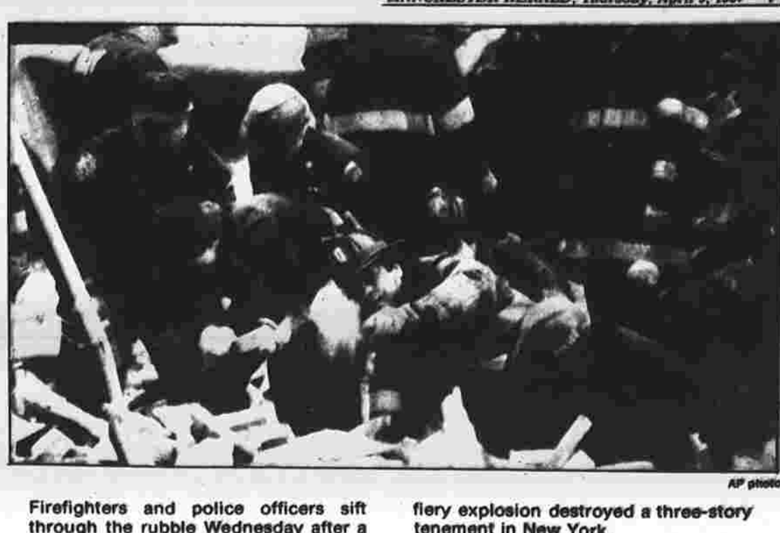
Firefighters and police officers sift through the rubble Wednesday after a fiery explosion destroyed a three-story tenement in New York.
